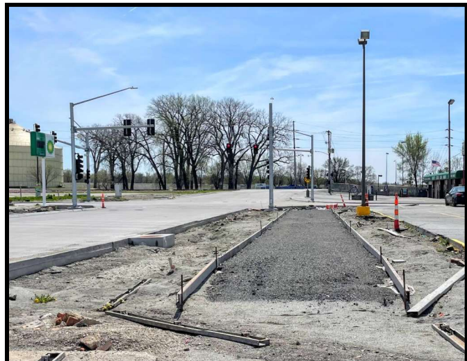
Trail Under Construction Along Warren Street
