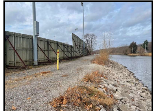
Existing gravel trail behind Bruner Field that is to be paved
