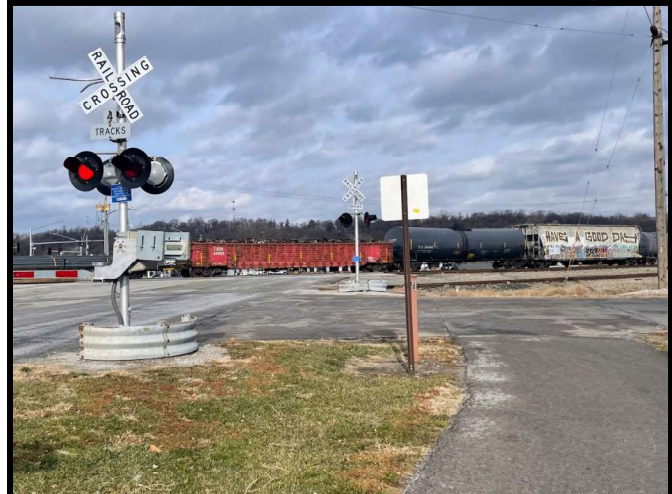
Proposed Location of Trail Crossing of Railroad Tracks
