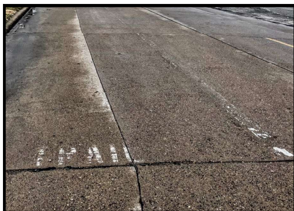
Pavement Marking Delineating the On-street Trail
