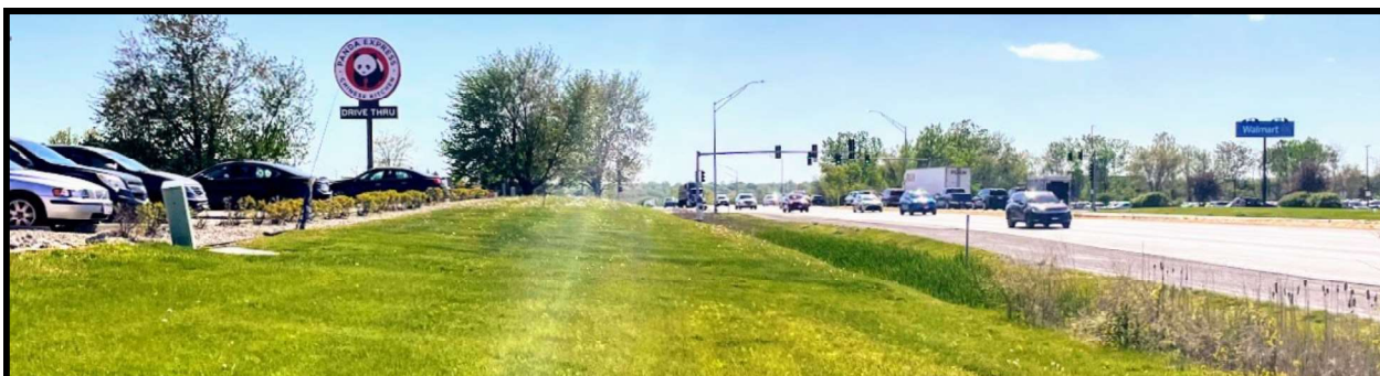
Looking southwest along U.S. 61 Drive from proposed trail alignment, at the U.S. 61/Allsteel/Walmart Driveway Intersection
